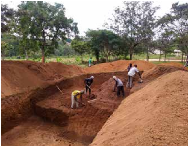
Digging the hole for the new water tank by hand.
